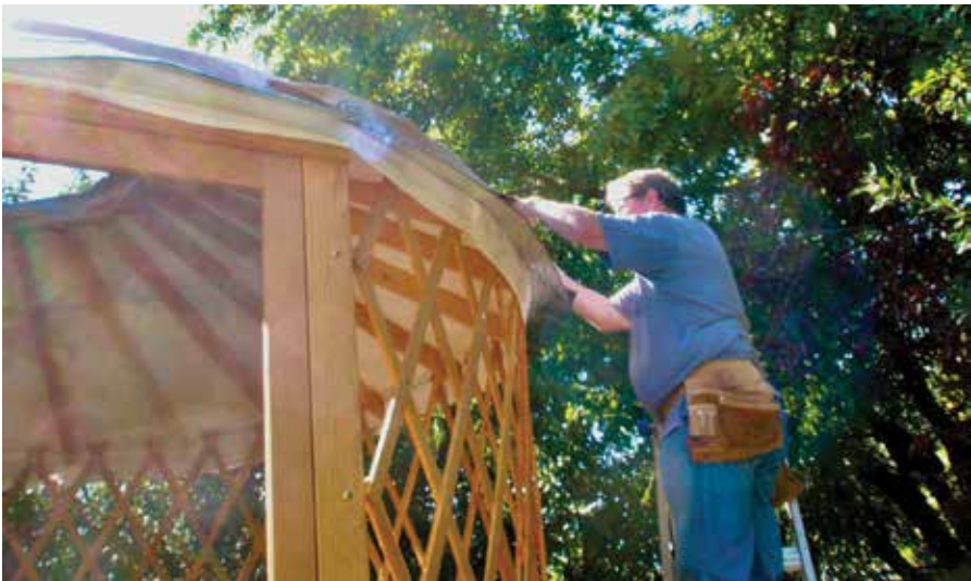
FIGURE 53: Rainbows and dharma wheel mandalas appeared as yurt was being constructed.
